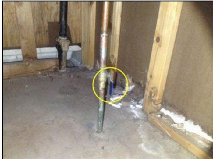
Main water shutoff valve behind water heater
