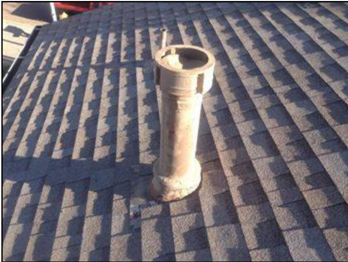
Metal B-vent - furnace & water heater
