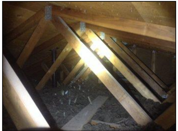
Trusses - upper attic structure
