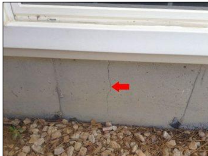
Typical minor crack
