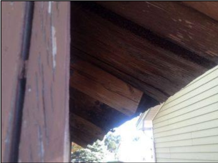
Rot - shed soffit (due to no gutter)
