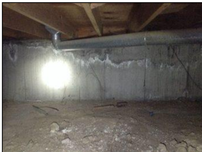
Efflorescence
