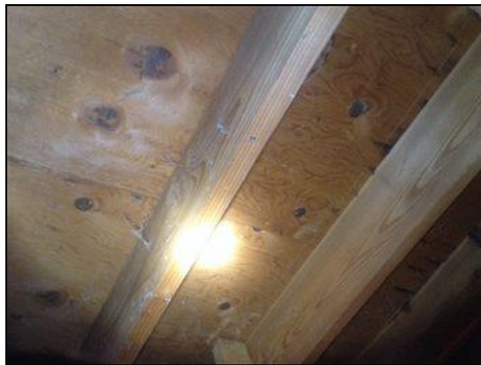
Joists, plywood sub-floor
