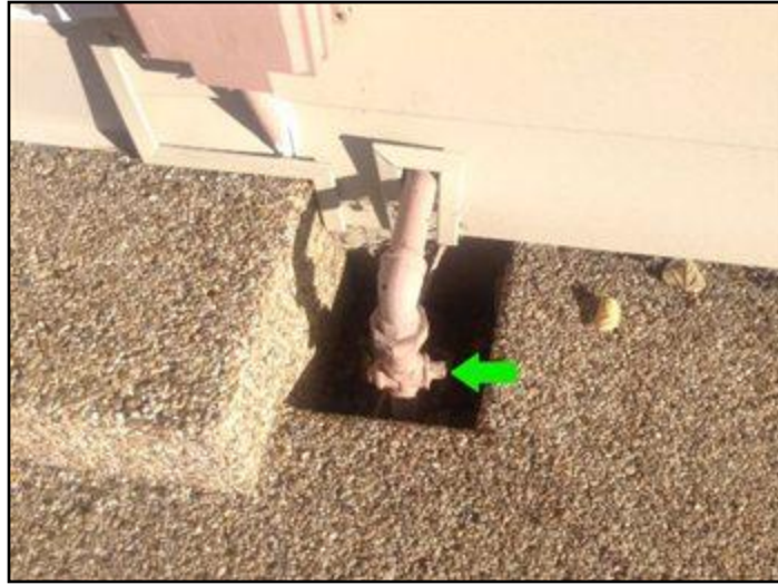
Exterior gas shutoff valve
