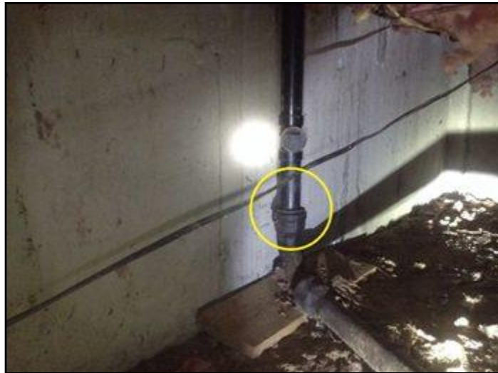
ABS connects to Cast Iron
