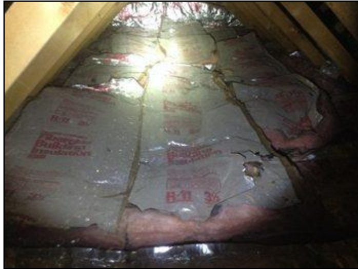
Glass fiber batts - lower attic
