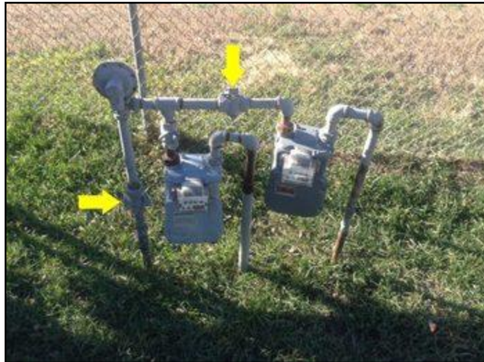
Gas shutoff valves + Meter
