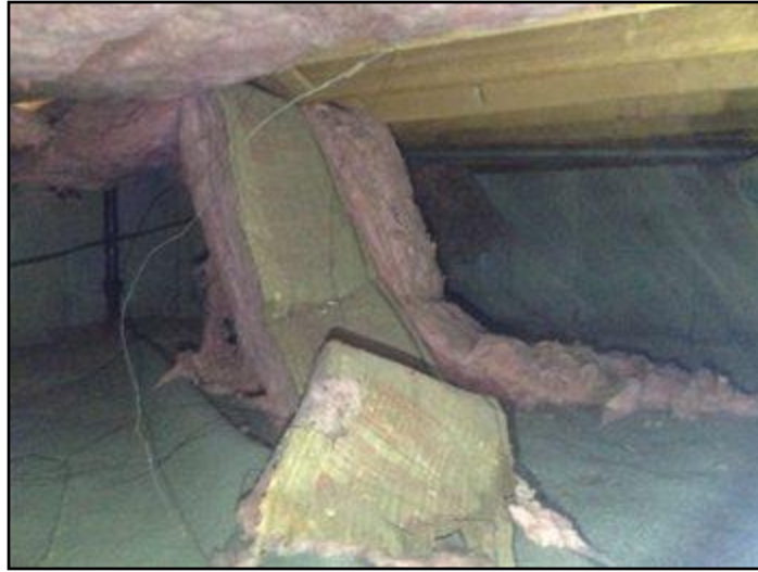
Gaps or voids, fallen insulation
