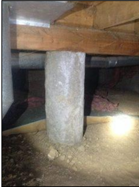
Wood beam, concrete columns
